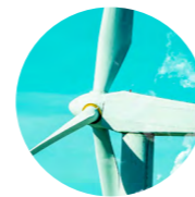
India Power project
